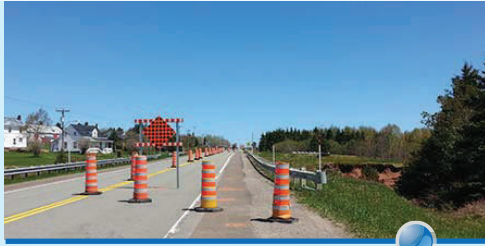
Circulation reduced in Shigawake due to landslide
