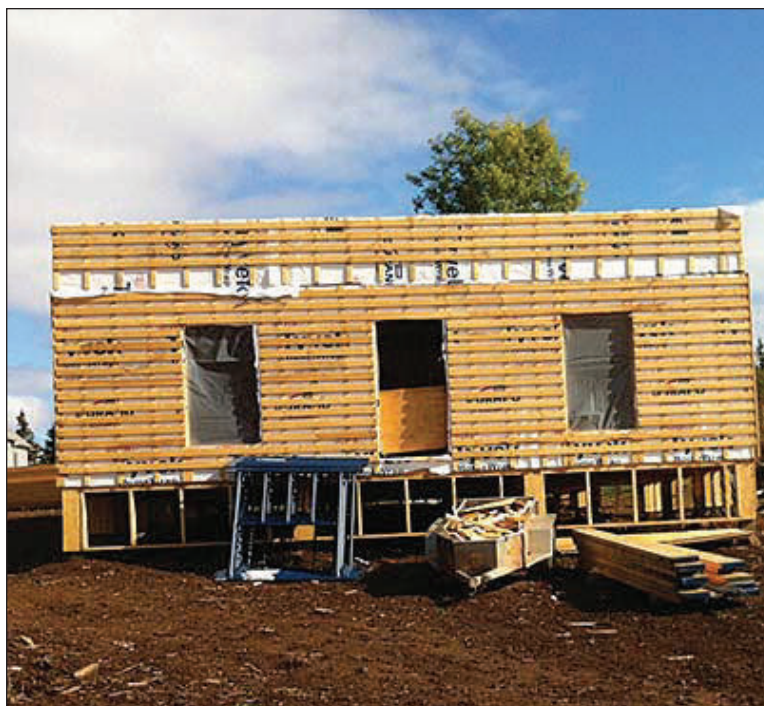
Construction of Paget House.
