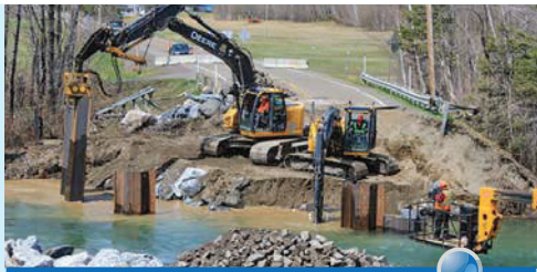
Work progressing at Trout Brook
