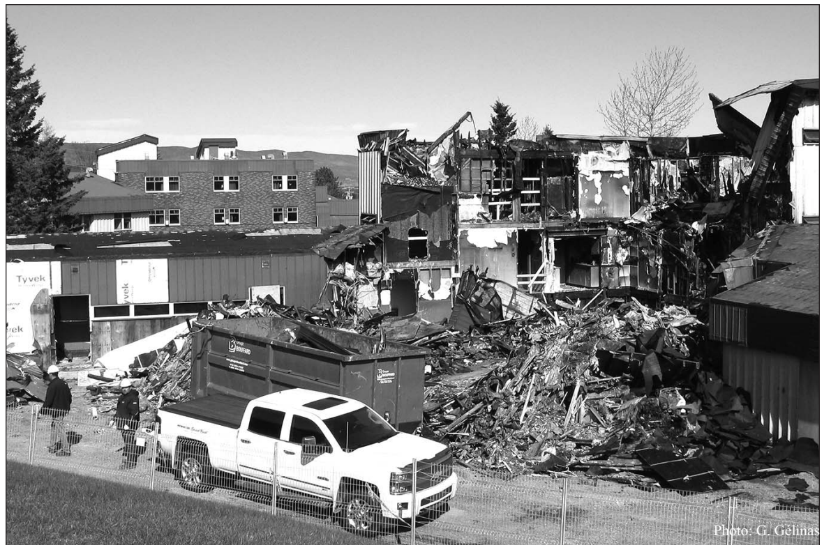
The St-Jean Pavilion of the residence, which burned on May 16, was being demolished when the SPEC visited on May 24.
