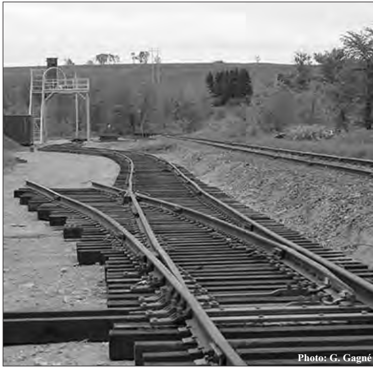
The Nouvelle transshipment terminal should be up and running before the end of June. The contractor is KLN.
