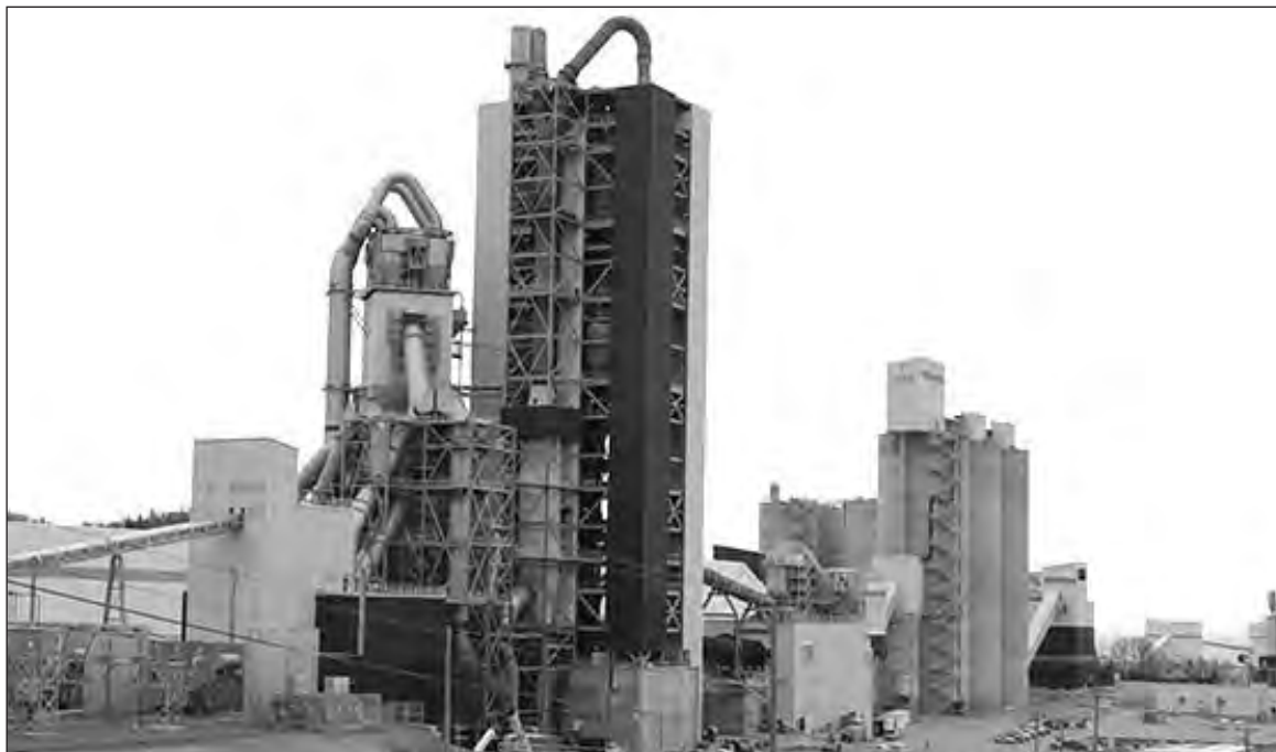
The refinancing of McInnis Cement will take the form of new investments, to add two silos to the Port Daniel plant and a rail freight yard.
