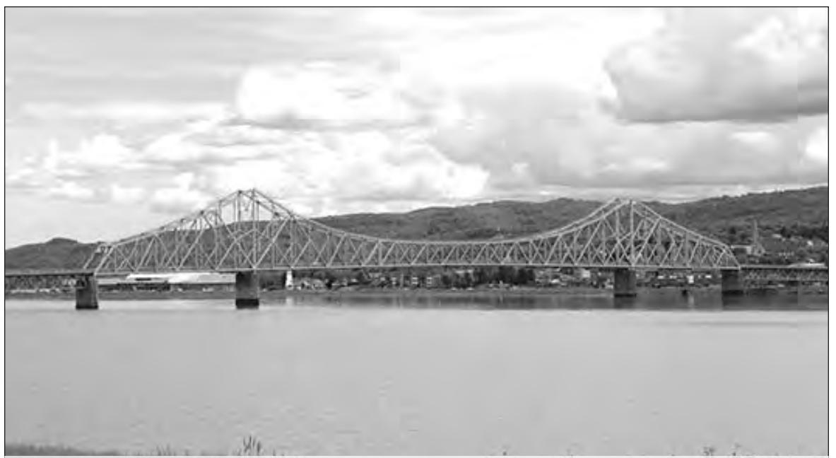
The J. C. Van Horne Bridge was inaugurated 58 years ago. For the moment, Supply and Public Works Canada cannot specify when it was last upgraded.
