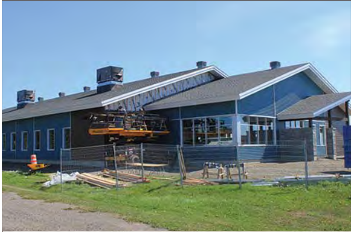
The exterior of the new building is almost finished. The interior should be ready by December.
