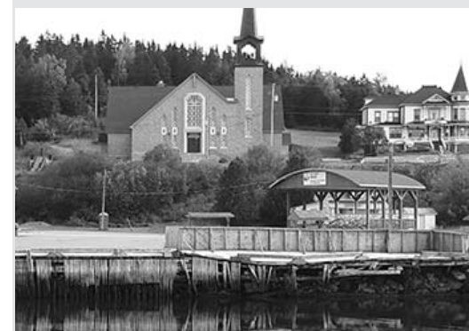
The wharf protects the tourist kiosk and public area in Port Daniel. Photo: N. Sergerie
