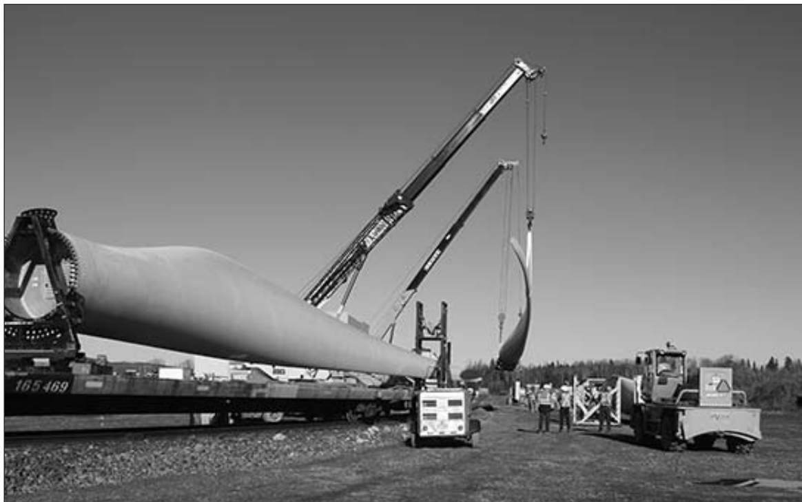
LM Wind Power must send its blades by truck between its York industrial park and New Richmond, where they are transferred to railcars.
