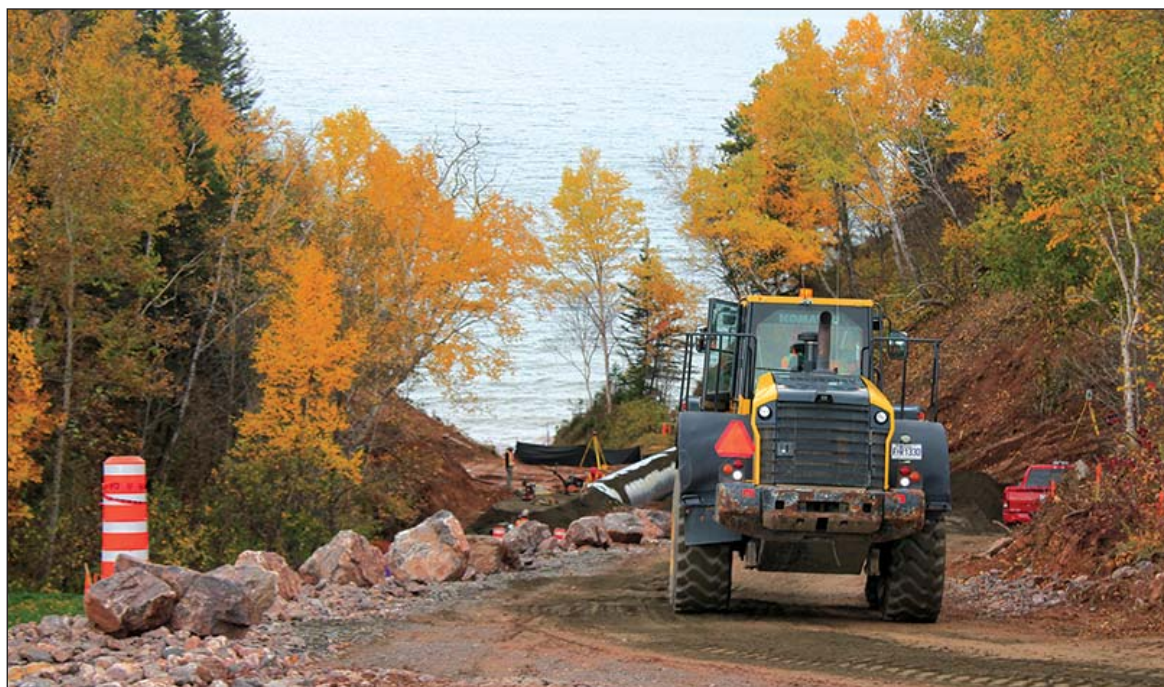
The Ruisselet Bridge is already gone and a new structure will be operational in the fall of 2021.
