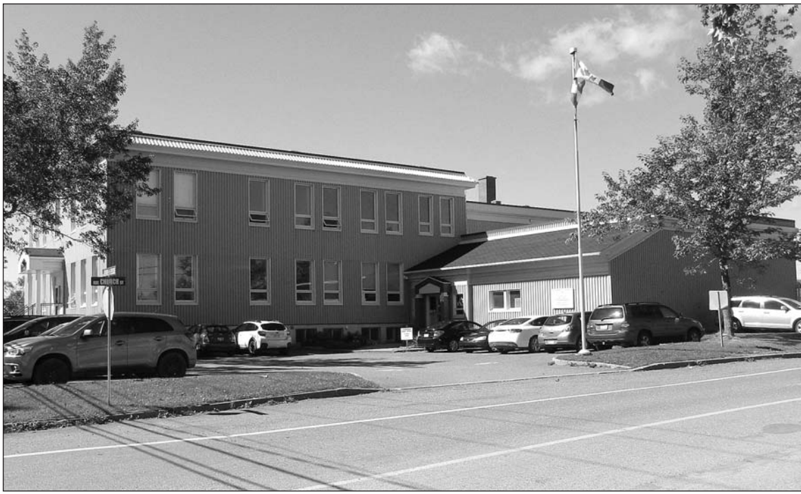
The presence of mold forced the closure of New Carlisle High School, effective on November 4, although the previous day was called a pedagogical day at the last minute to adapt to the situation.
