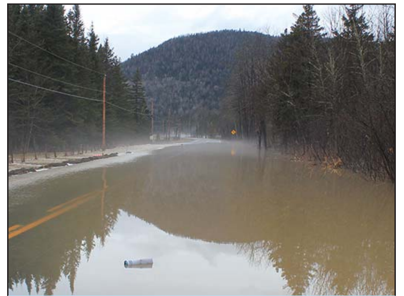
Road 299 sustained heavy damage, mostly around the 12.5-kilometre point, where the White Brook bridge was destroyed. The road was, nevertheless, closed around the 7th kilometre, for safety reasons, as the water of other brooks was passing vigorously on the pavement.
