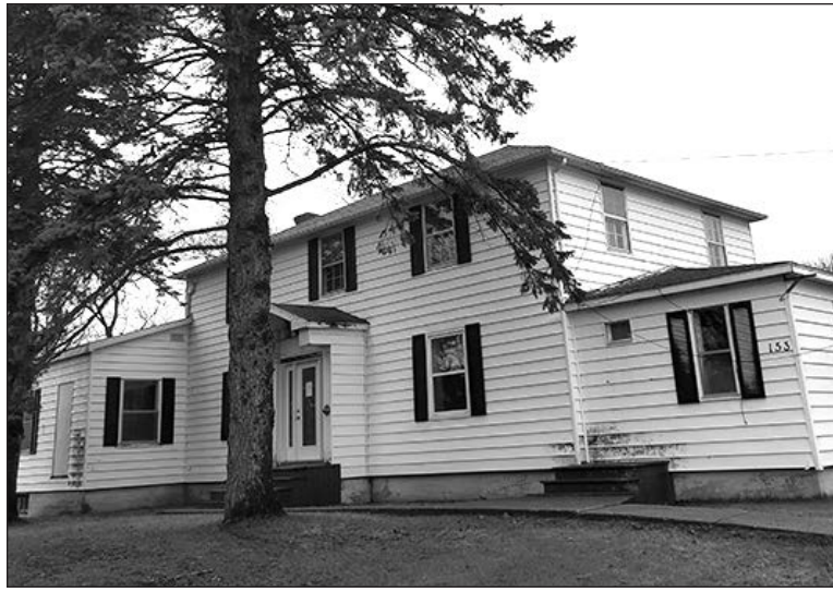
CHNC's building used to house the family of its founder, Charles Houde, and the radio station. The building no longer has the functionality required for the radio station.
