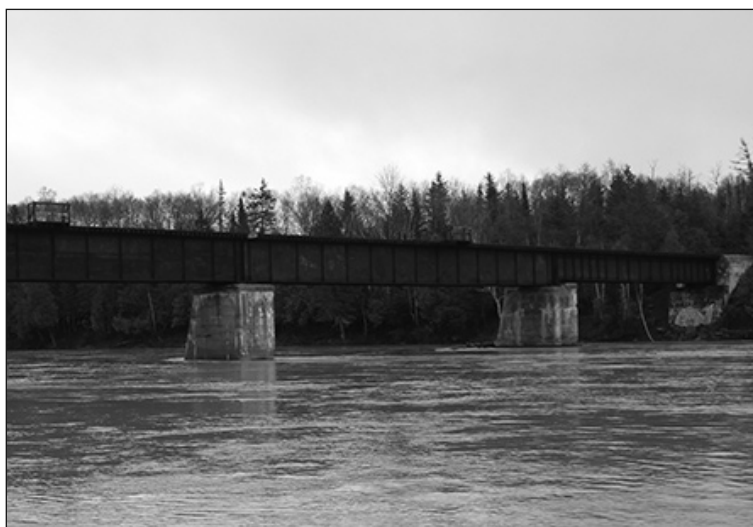
The Bonaventure River bridge will be repaired by Groupe SEMA, following a bid of $6,539,854.
