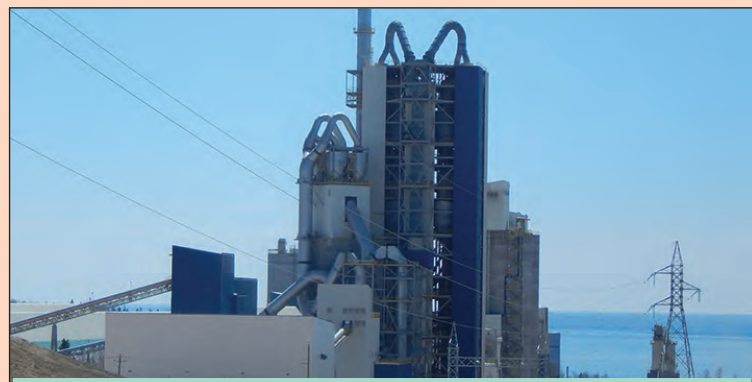
Ciment McInnis responded on August 31 to the Ministry of the Environment on dust emissions since 2020.
