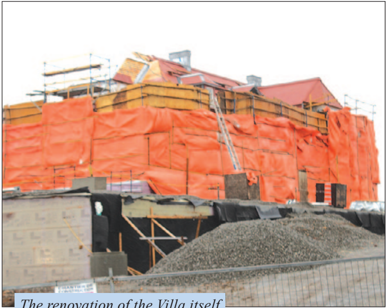
The renovation of the Villa itself took place primarily in 2023.
